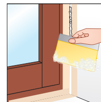
Finish the sealing with a wet spatula
